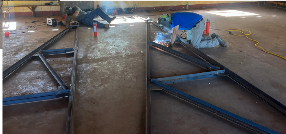
Welding the trusses
