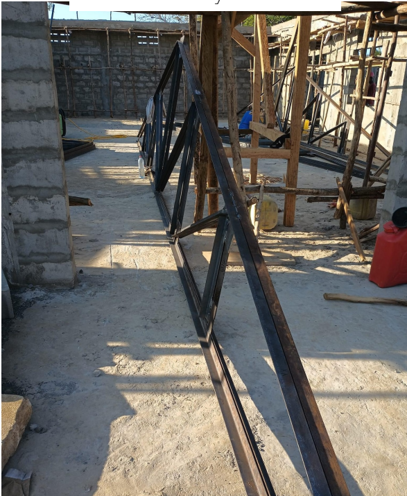
Holding the truss steady while the welders attach it.
